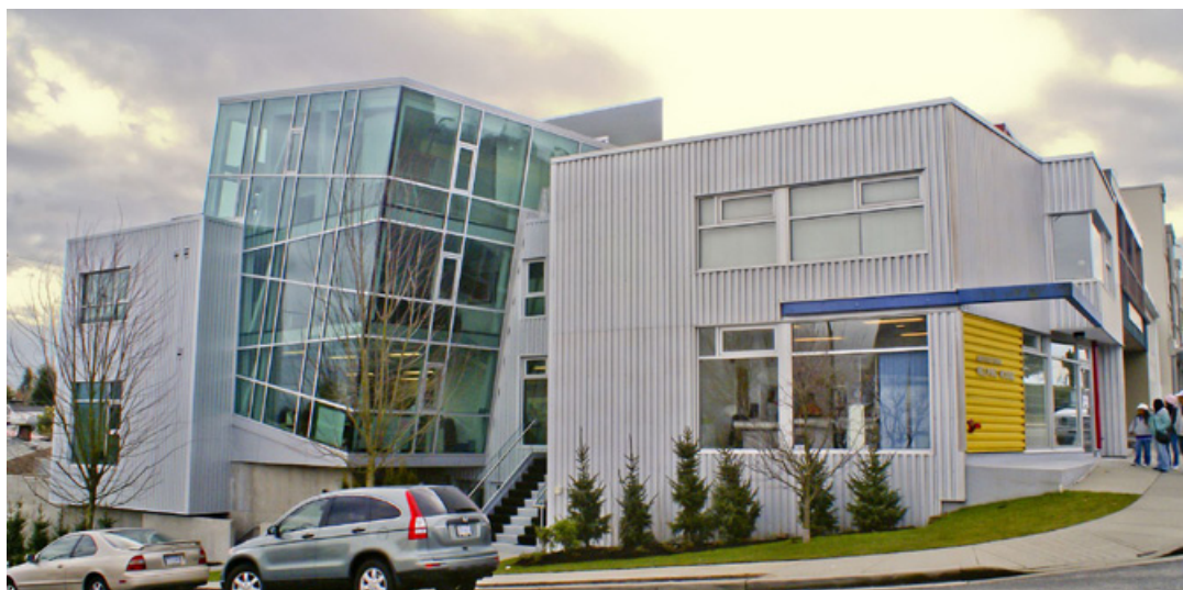
Expansion of the Multicultural Helping House (Vancouver). Photo courtesy of Infrastructure Canada.
