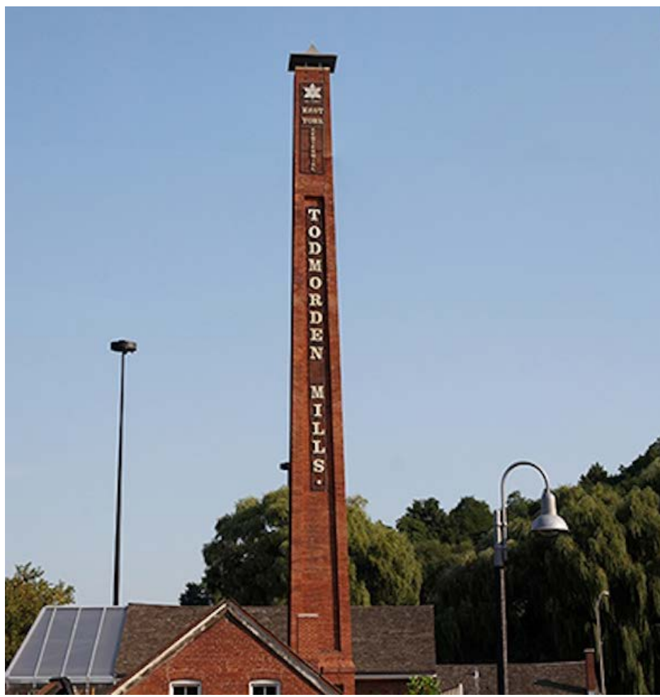
Photo: Papermill Tower – After
